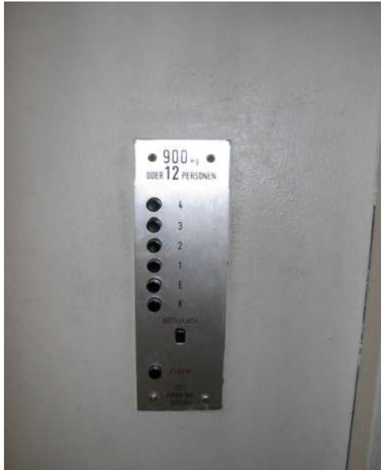
CS Building in Saarbrücken
