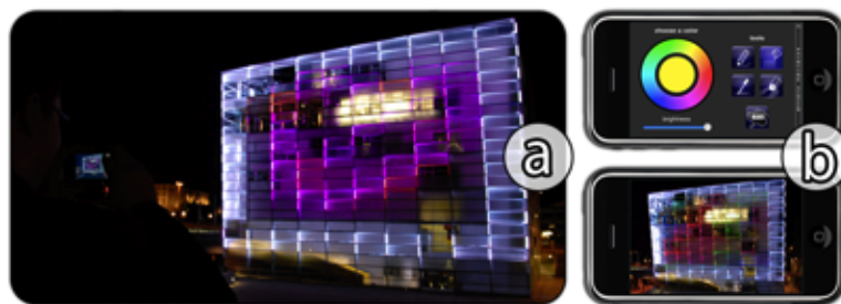
Figure 69. (a) Users can interact on the entire façade using their mobile device. (b) They choose their individual color and tool and apply these to the façade directly through live video (Boring et al., 2011). 66
