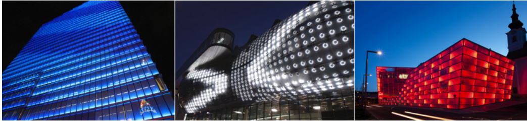
Figure 64. Light emitting media façades embedded into contemporary architecture that may display (remote) interactive content (from left): Dexia Tower, Brussels, Belgium, Kunsthaus, Graz, Austria and the ARS Electronica Center in Linz, Austria (Wiethoff and Gehring, 2012). 60
